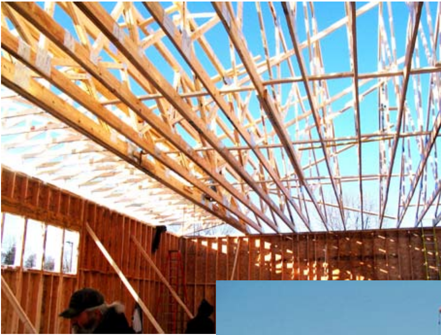
Warehouse addition - Setting trusses
